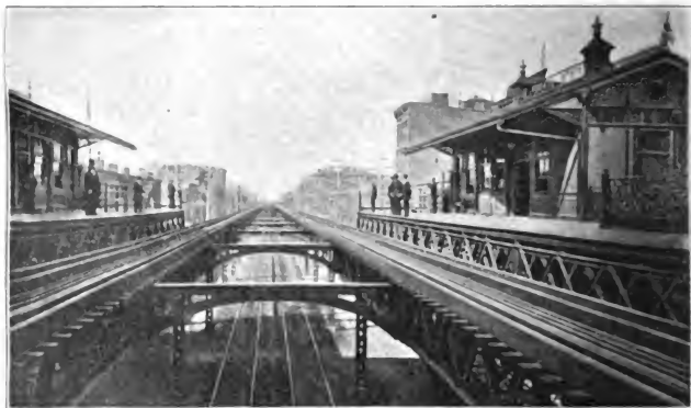
THIRD-AVENUE ELEVATED RAILROAD, LOOKING NORTH FROM 9TH-STREET STATION, BUILT BY A. R. WHITNEY & CO.
